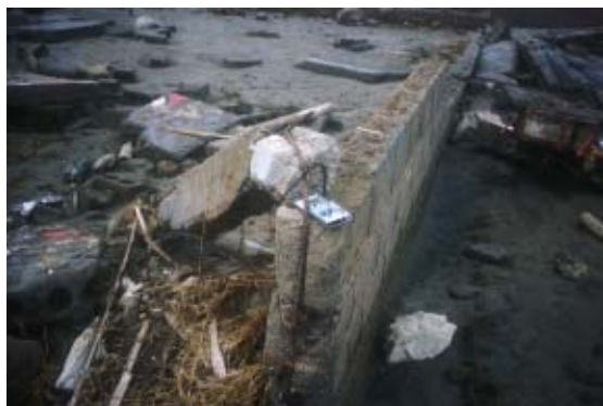
Figure 6.19 Reinforcing bars bent by tsunami.
