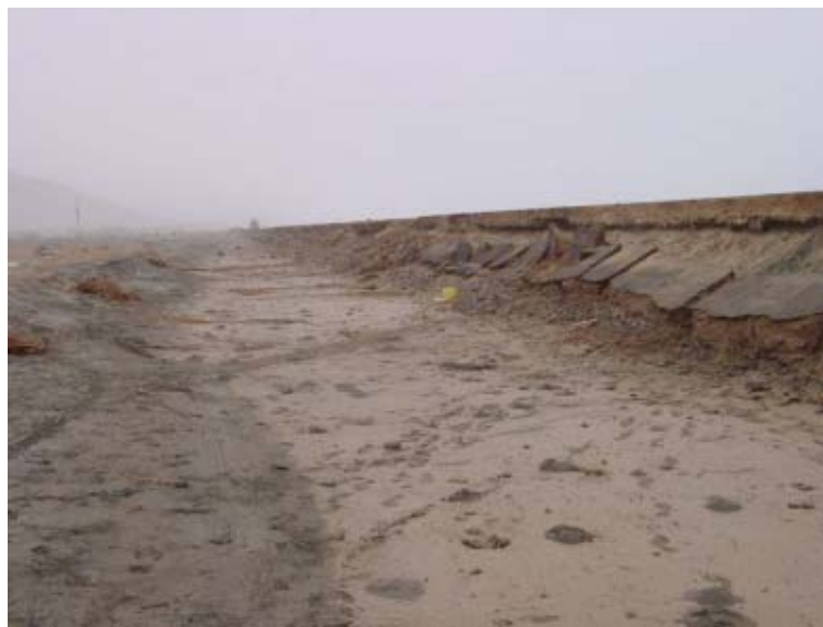
Figure 6.5 The erosion of the beach of La Punta, Camana
